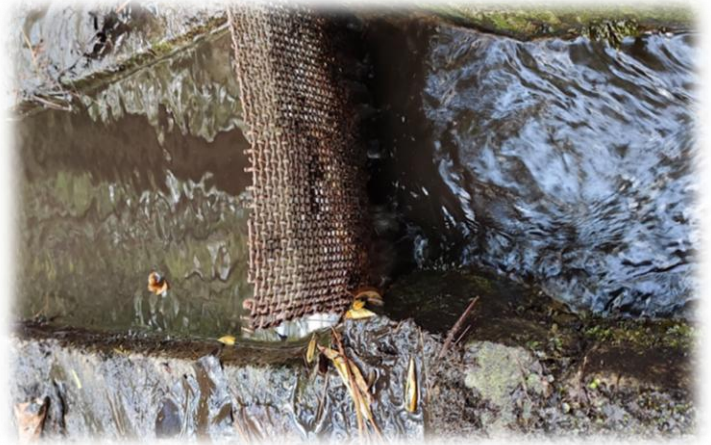
Figure 5: wire mesh used to remove debris to reduce turbidity in some rural water supply
