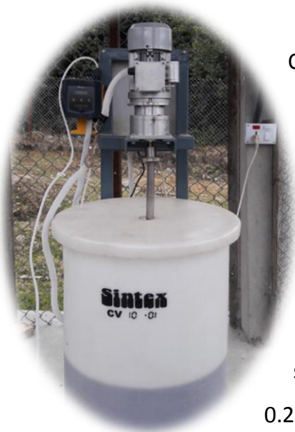
Figure 7: Chlorine dosing machine used in some WTP
