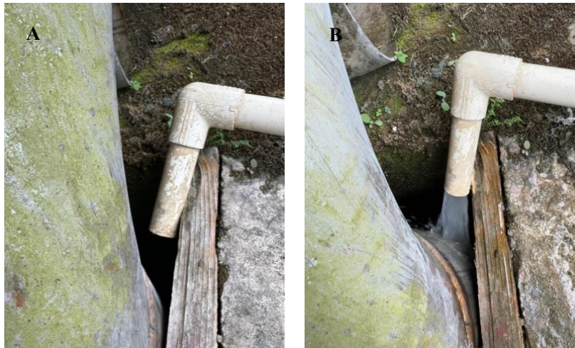
Figure 1 Inappropriate chlorine dosing practice (A. Before adjusting chlorine dose and B. After adjusting chlorine dose)
